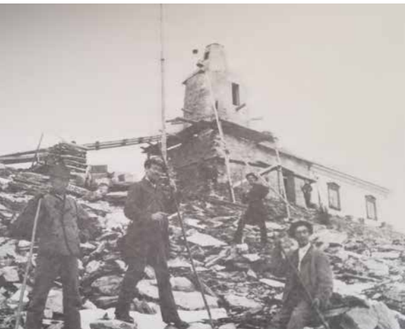
Bauarbeiten am 24. August 1886 Construction work on 24 August 1886
